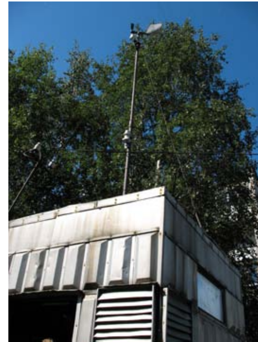
Monitoring post in Severodvinsk
