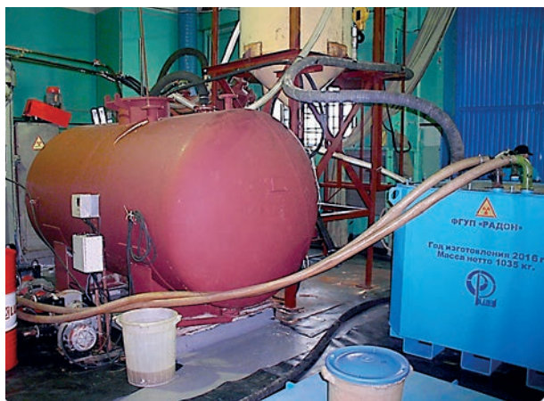
Fig. 4. IER impregnation with polymer binder in a KMZ container
